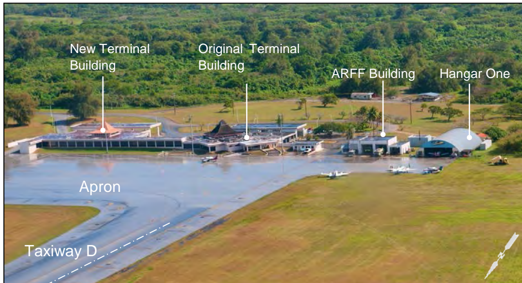
Photo 2.1-15. Airside Access to the Passenger Terminal Building (Looking South)
