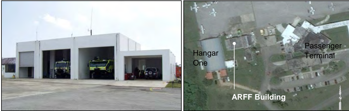
Photo 2.1-16. Aircraft Rescue and Firefighting Building
