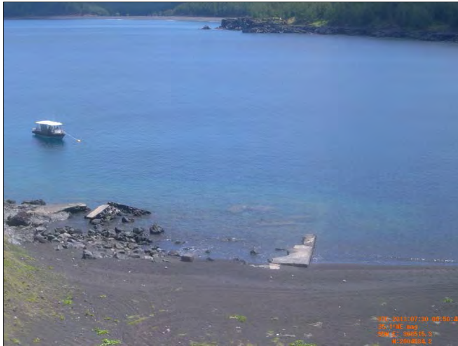
Photo 2.2-7. View of Pagan Pier in Current Condition
