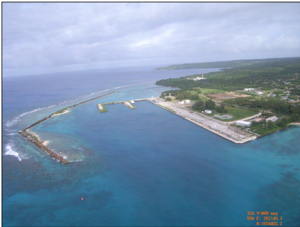
Photo 2.1-23. Overview of the Port of Tinian
