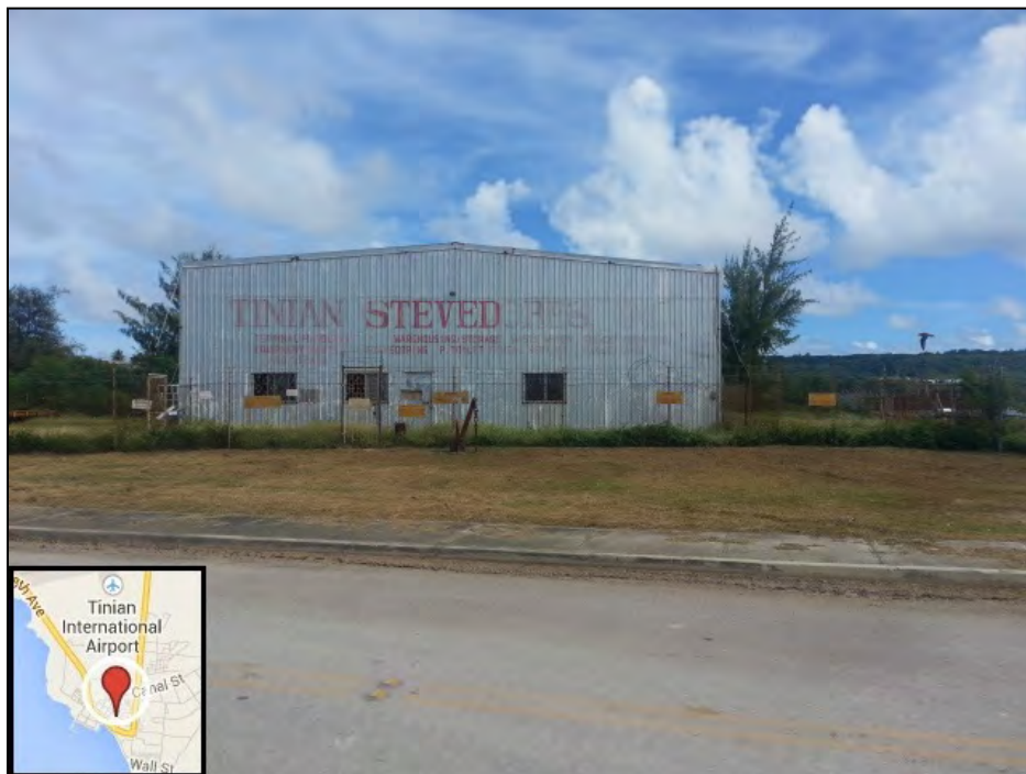
Photo 2.1-13. Example of Tinian Existing Sidewalk in San Jose Near Port
