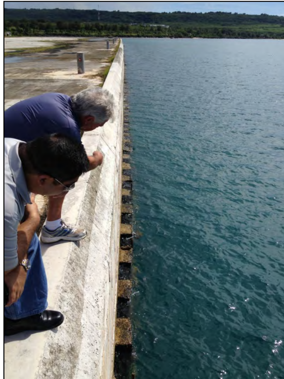
Photo 2.1-27. Main Wharf of Port of Tinian (note sheet pile along waterline)
