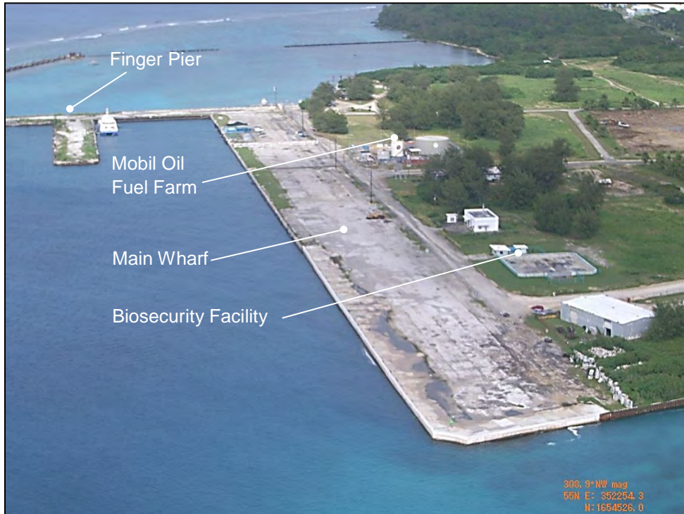
Photo 2.1-25. Port of Tinian Main Wharf and Port Facilities
