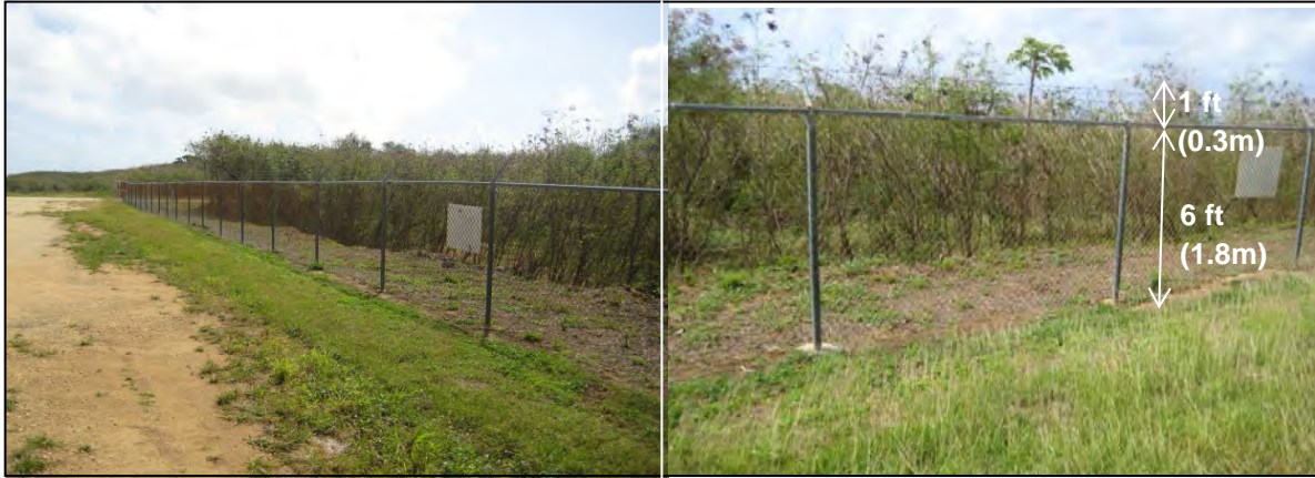
Photo 2.1-18. Existing Security Fence
